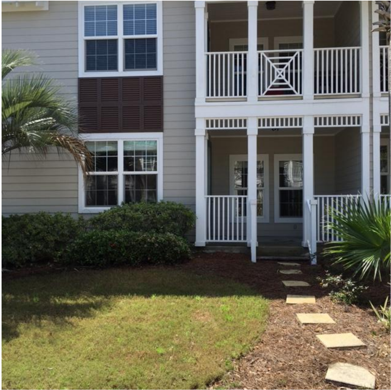
Front entry to bottom level unit.
